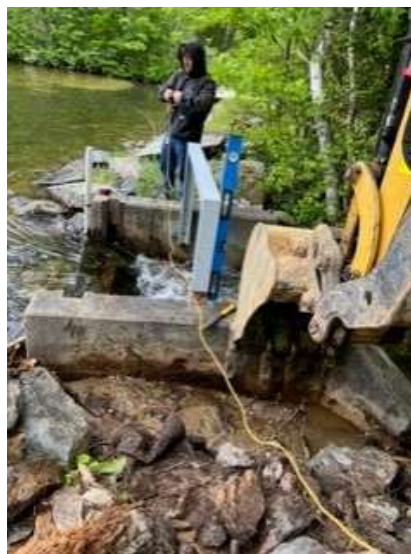
Repair of leaning spillway
